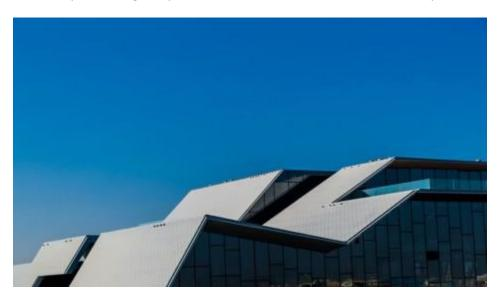
The roof is cladded with ceramic and steel tiles following a geometric pattern. Colorful and shining by day time, it will be lit up with LEED tricolored projectors by night; it is an installation by CAI light.
