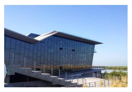
Spaces open up from a folded crossed cut slab: the slope of the folded roof starts from the entrance and reaches up to the highest point where it leads to terraced/belvedere spaces for looking out the sea.
