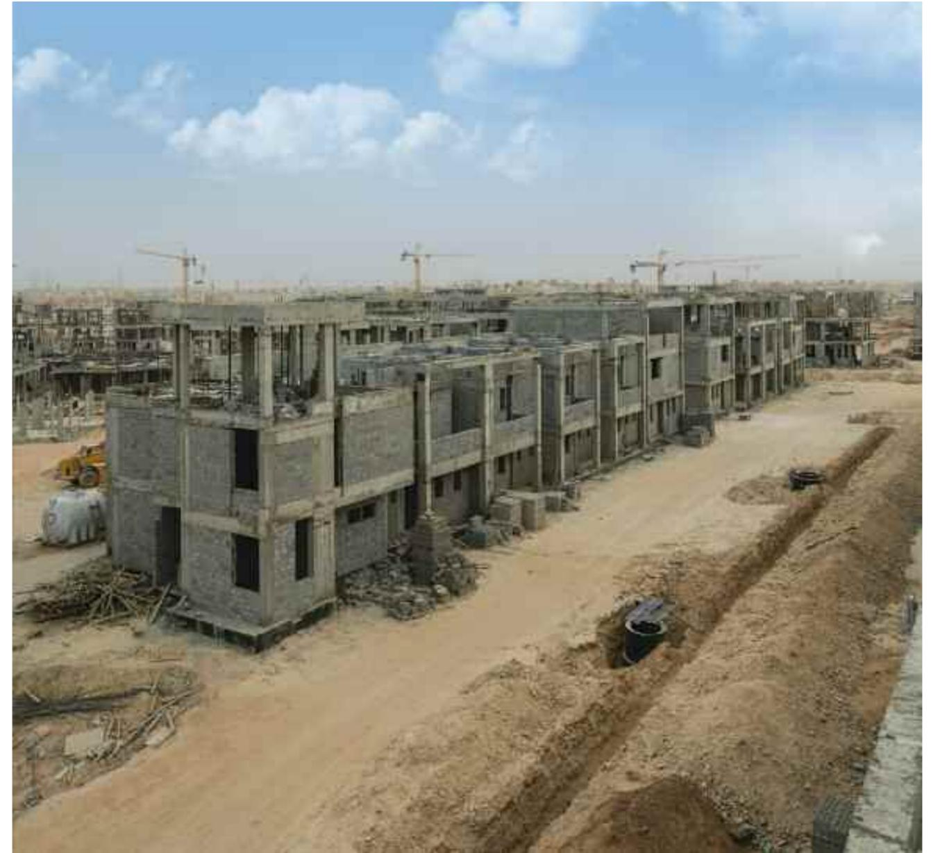
Following excavation and grading, 95 percent of the structural works for the villas and apartments have been completed to date and mechanical, electrical, and plumbing and finishing works have started in several locations. A mock-up villa has been constructed to serve as a guide for finishing the rest of the site.
